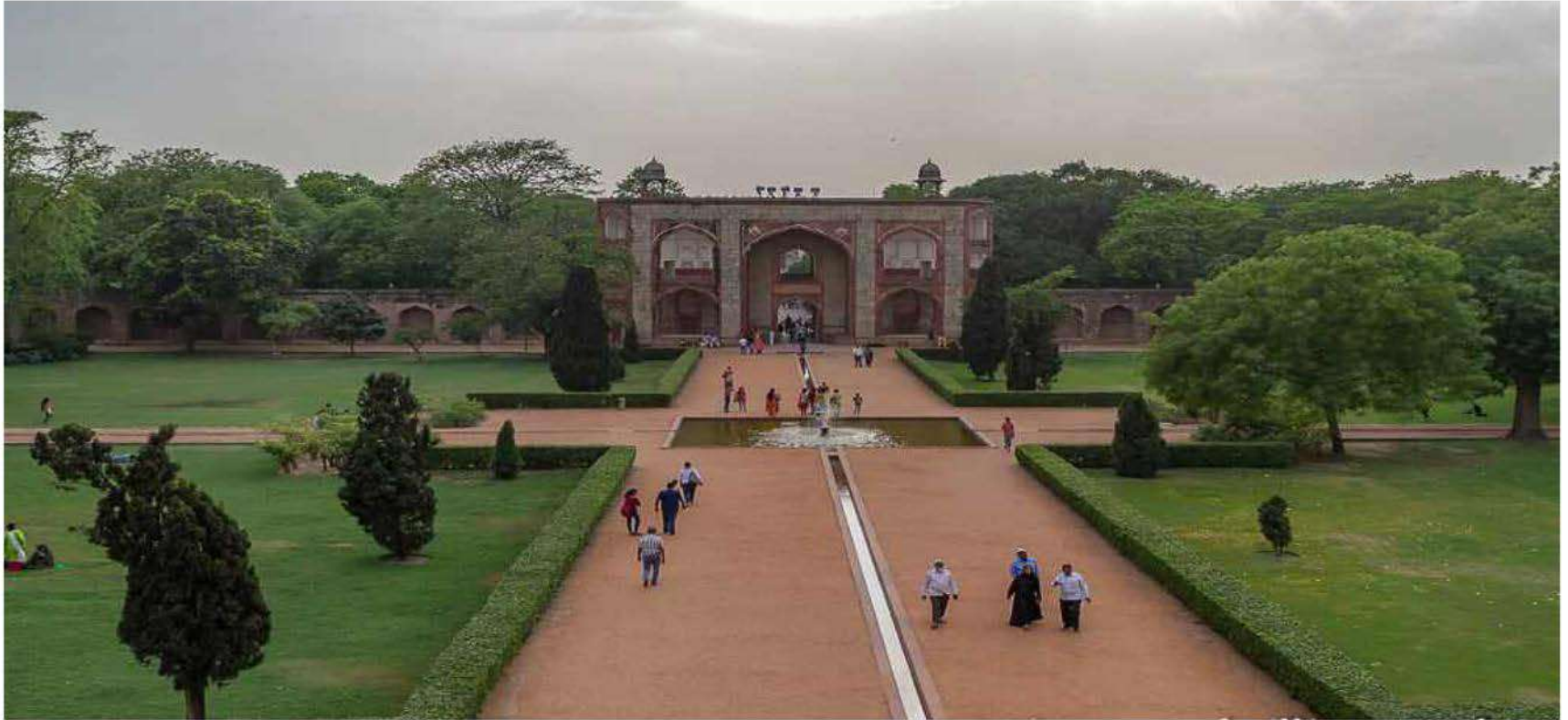
The west gate, the main entrance. The char bagh gardens with channels of water and fountains
